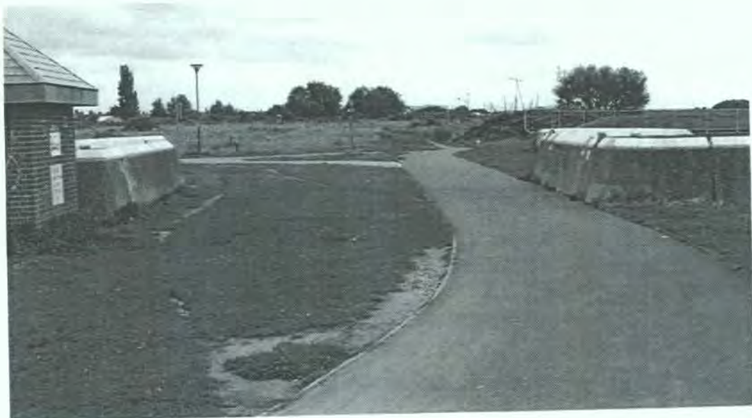
Figure 3.1: Nar Ouse Outfall Sluice and Existing Pedestrian/Cycleway
